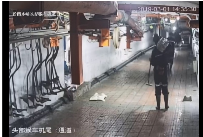
Carrying objects when field workers are on the lift chair
