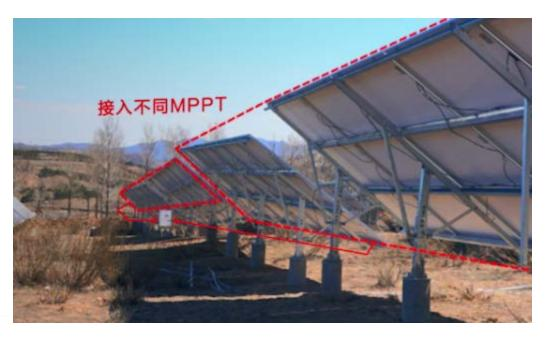
2 PV strings per MPPT to Reduce the impact of PV string shielding and different orientations, +3% more generation
